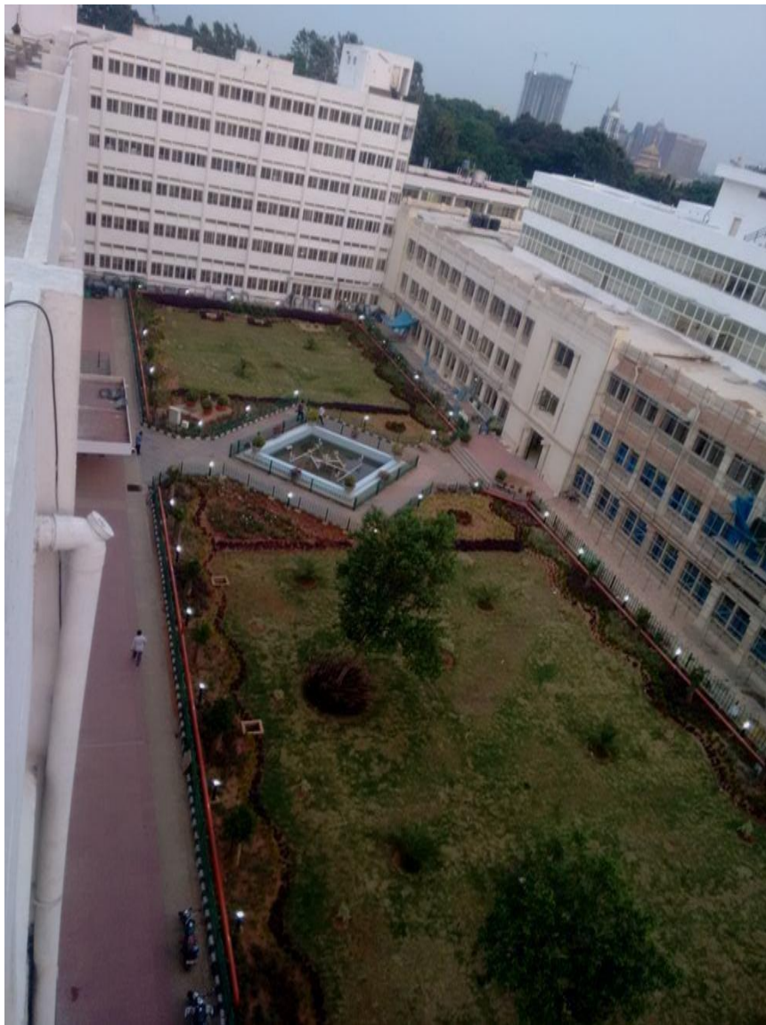
Fire Fighting System at Legislative House, Bengaluru. IC India Private Limited, Bengaluru.
